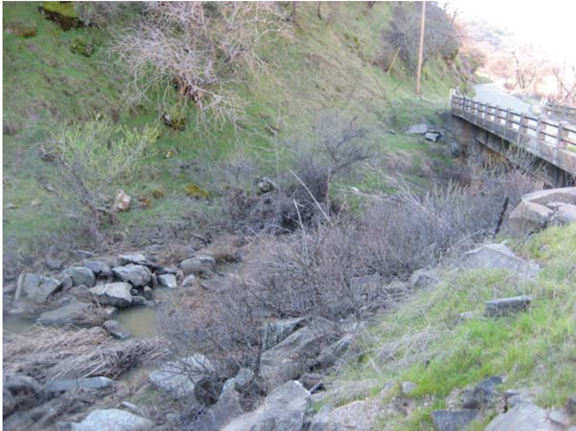
Stone Corral Creek Immediately Downstream of the Proposed Sites Dam Location (Looking Upstream) (2/23/2011)
