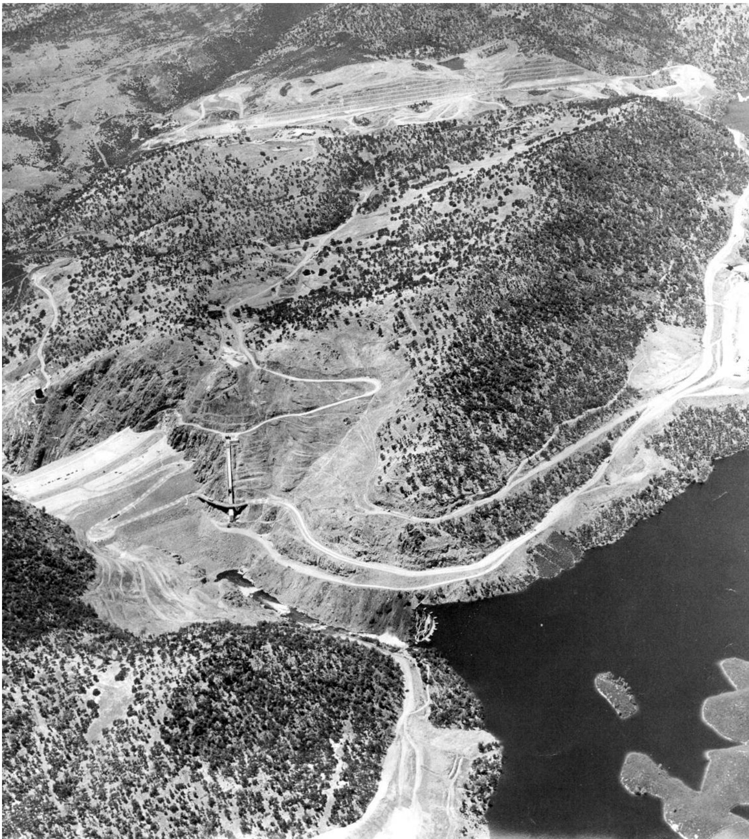
Water spills over the old Melones Dam, built in 1928, in the foreground, as New Melones Dam takes shape in this June 2, 1978 aerial photo. At top, the new spillway is being cut into mountain. The project first approved by Congress in 1944, but not completed until the late 1970s. It was the last major dam built in California. Forrest Jackson Jr. FRESNO BEE FILE
