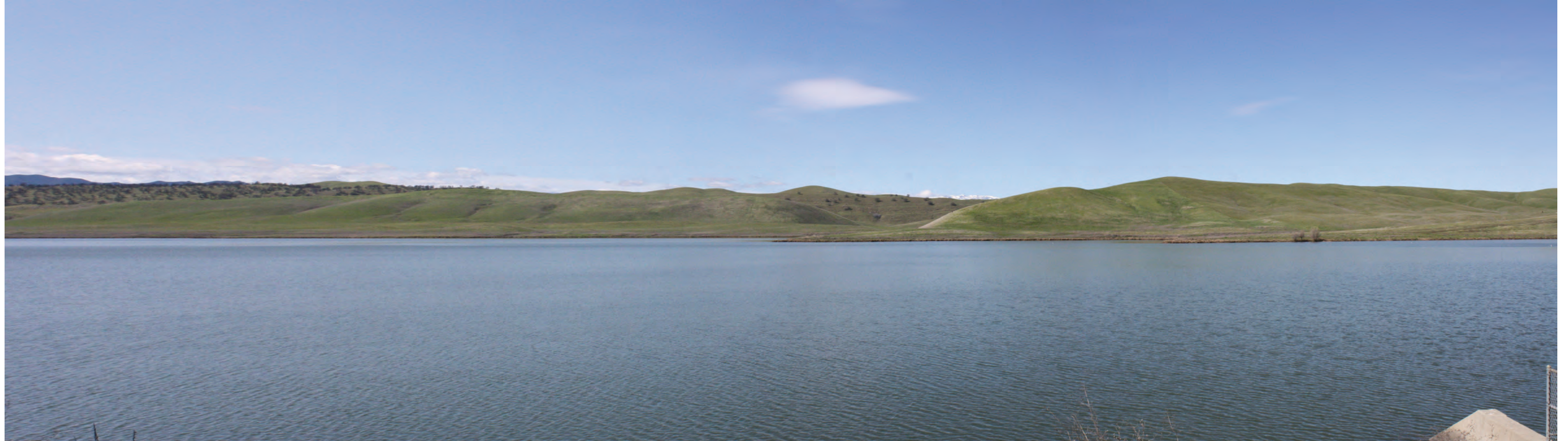
Photo 21: Looking west at the existing Funks Reservoir toward the Field Office Maintenance Yard location (to the right of center of photo) from the downstream side of Funks Reservoir near Funks Creek and the Funks Dam Spillway.
