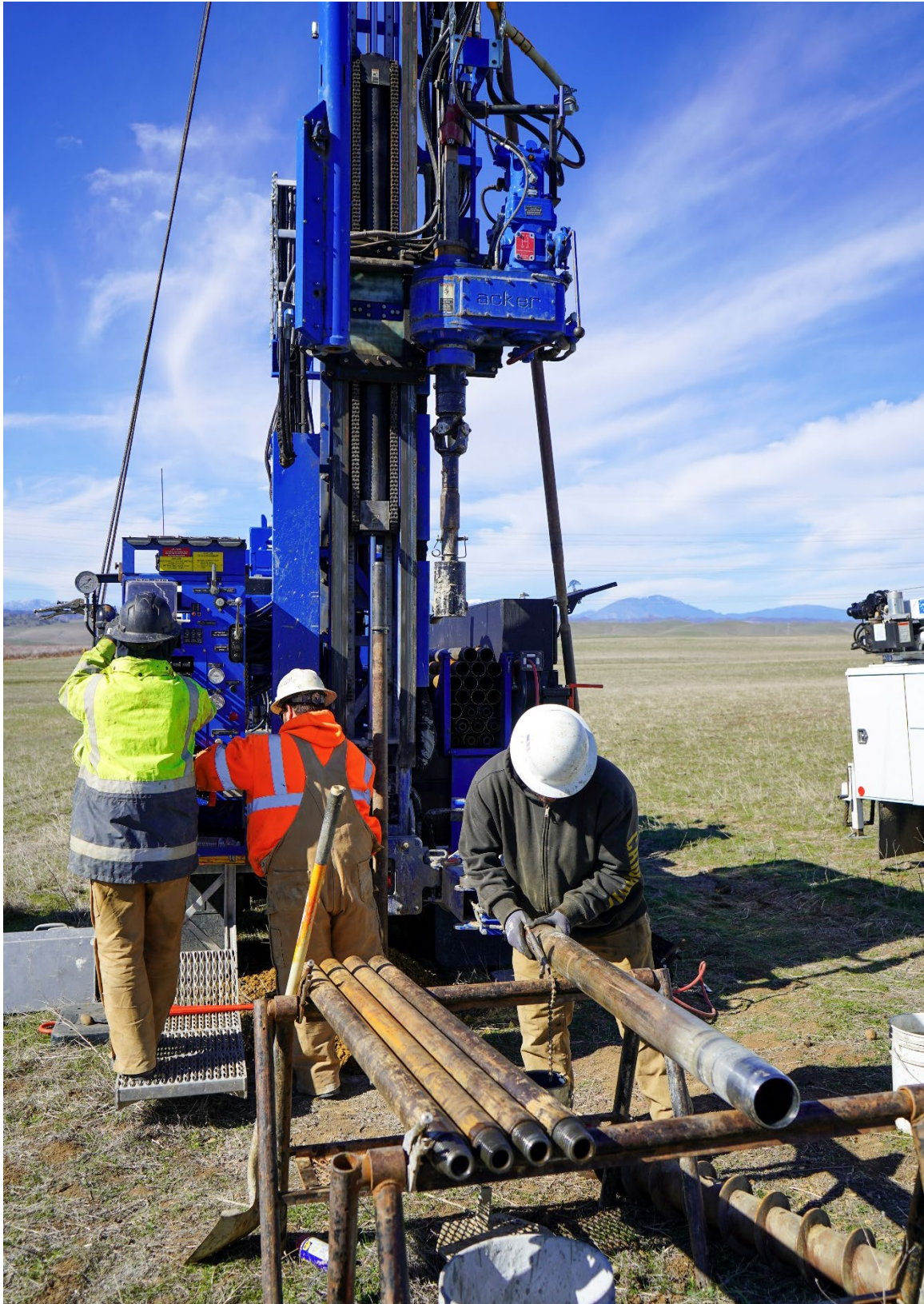
Photo 6 – Representative photo of drill rig crew collecting core samples.
