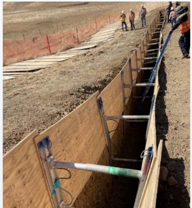
Figure 3. Fault Trench Excavation for Sites Project, October 2023.
