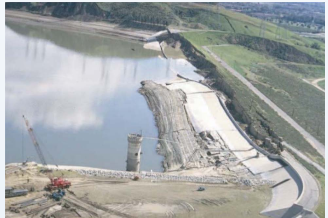
Figure 1. Lower San Fernando Dam after the San Fernando earthquake (1971). (Courtesy of the National Information Service for Earthquake Engineering, EERC, University of California, Berkeley)
