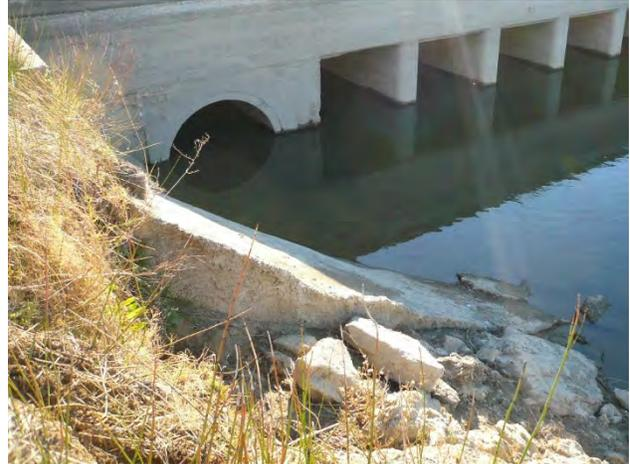
**Figure 20. Canal Bank Erosion at Western Side of Outlet**
