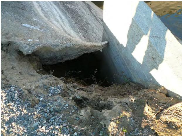
**Figure 17. Canal Bank Erosion at Eastern Side of Inlet**
