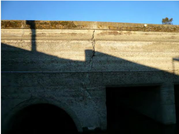
**Figure 28. Crack at Western Side of Inlet**
