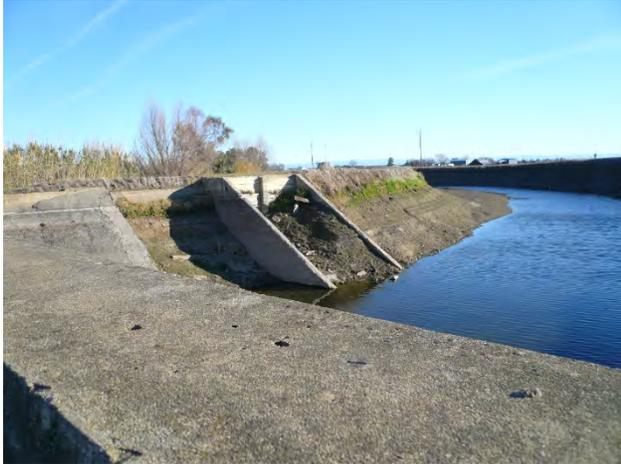
**Figure 19. Canal Bank Erosion at Western Side of Inlet**
