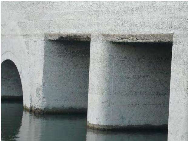
**Figure 21. Spalled Concrete**
