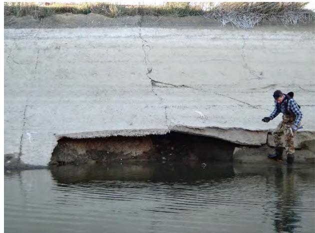
**Figure 18. Canal Bank Erosion at Eastern Side of Outlet**
