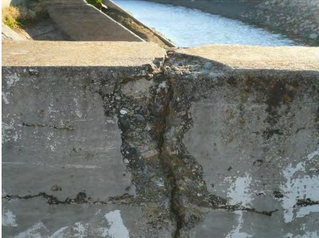
**Figure 26. Crack Through Guardrail Wall and Spalled Concrete**
