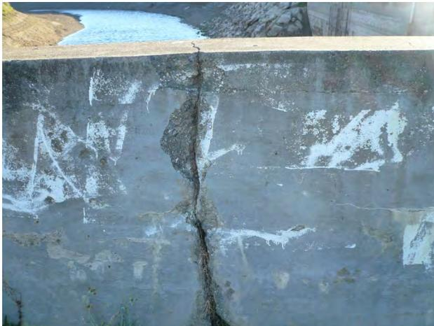
**Figure 24. Crack Through Guardrail Wall**
