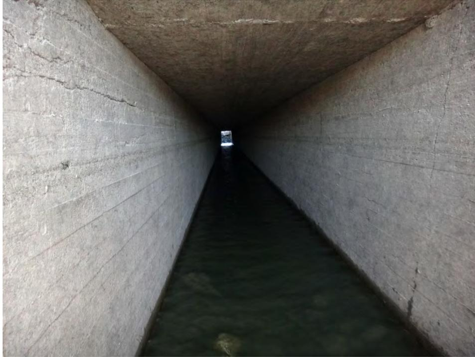
**Figure 10. Typical Siphon Bay from the Original Siphon Project**
