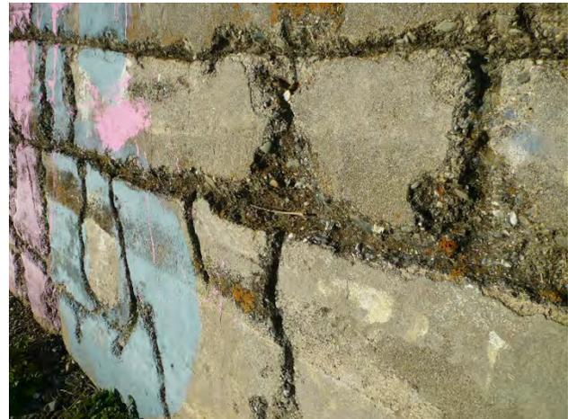
**Figure 25. Extensive Cracks at Guardrail Wall**
