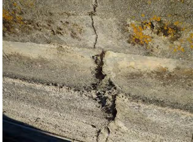
**Figure 27. Crack Through Guardrail Wall**
