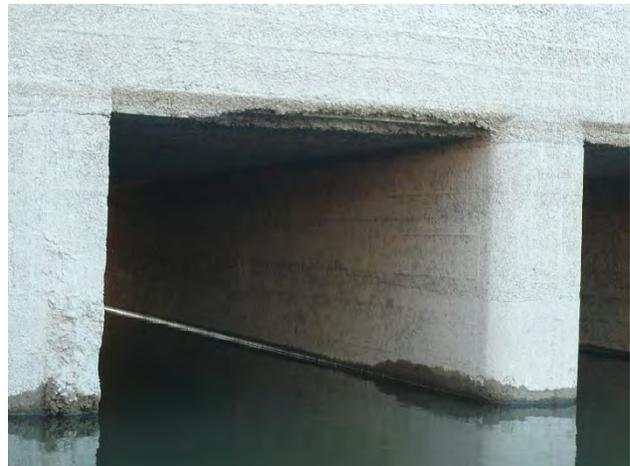
**Figure 22. Spalled Concrete**
