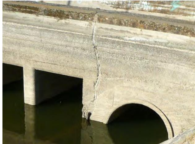
**Figure 29. Crack at Eastern Side of Inlet**
