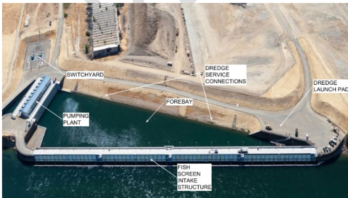
Figure 5. Aerial Photograph of the RBPP Forebay (CH2M 2013)
