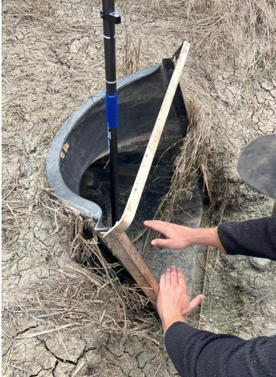
Figure 18. Rice Field Drainage Structure, with Flashboards Removed, Allowing Water to Drain into CBD
