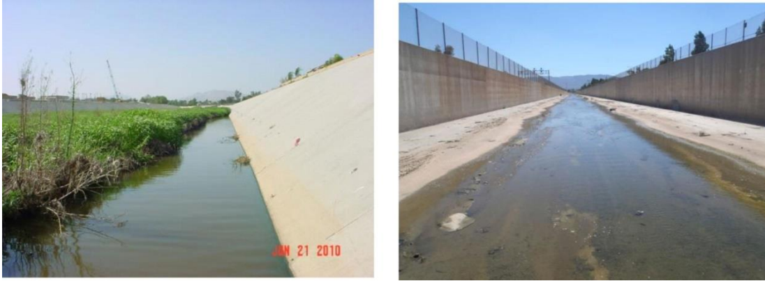
Figure 3. Two highly urbanized sites in the south coast, on the left with a natural soft bottom and on the right with a concrete bottom. Originally, the site on the left had an index score of 0.44 and the site on the right a score of 0.62, neither of which is an especially good score, but it was counter-intuitive that a site with a natural bottom would have a lower score than a completely concrete channel. After the “concrete correction” described in the text, the score at the site on the right was reduced to 0.35.
